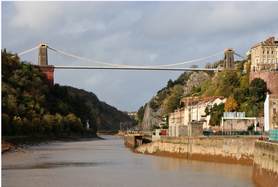
Figure 3.13: The Clifton Suspension Bridge, designed by Isambard Kingdom Brunel, spanning the Avon Gorge
